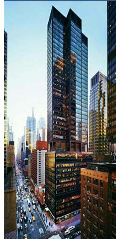
810 Seventh Avenue New York, NY Class E System Replacement
