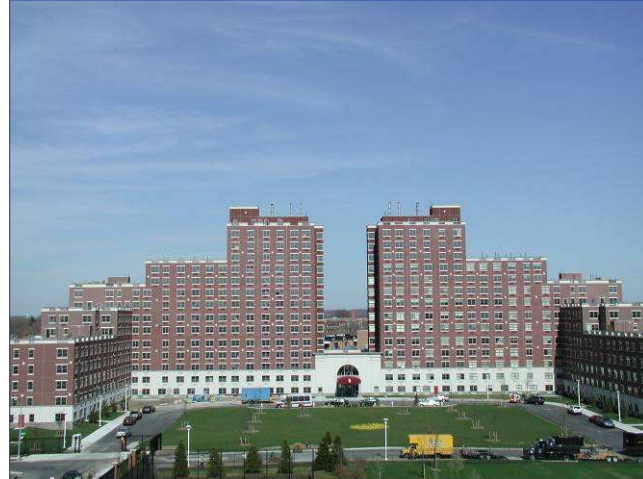
Kew Gardens Residential Complex - 550,000 sf
