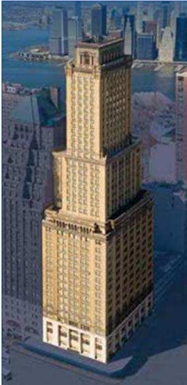
16 Court Street Brooklyn, NY Class E System Replacement
